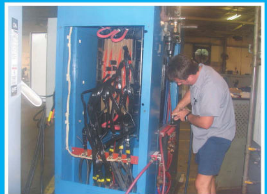
Transformer after being repaired
